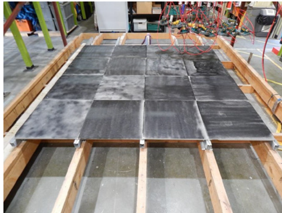
Figure 3. Installation of the paver system.
