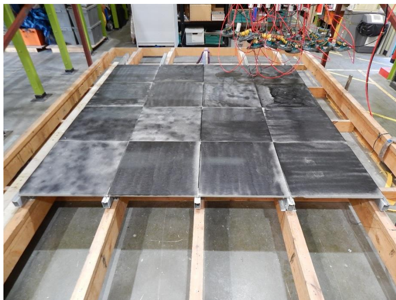
Figure 3. Installation of the paver system.
