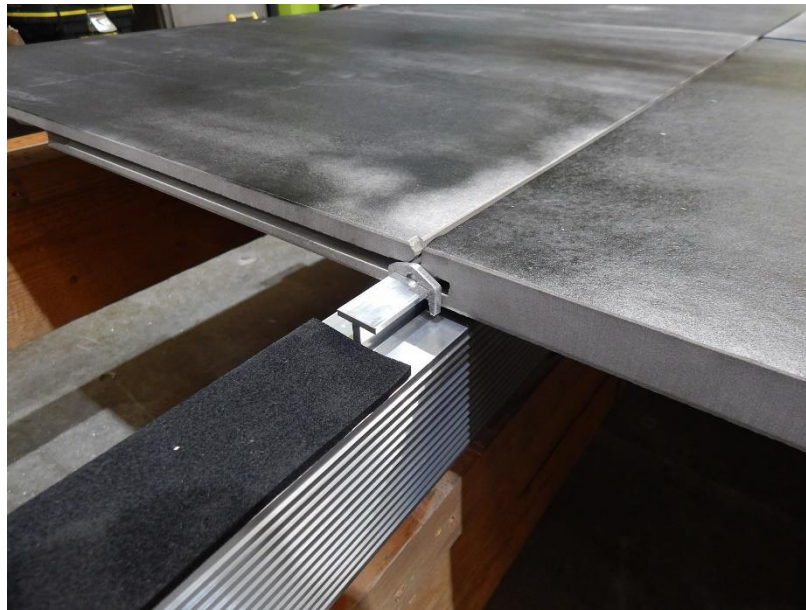
Figure 2. Close up of beam, J Clip, paver connection.
