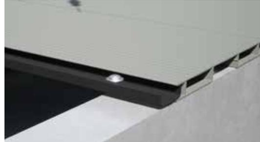
2. Take the next deck board and align onto the other side of the drainage channel.
