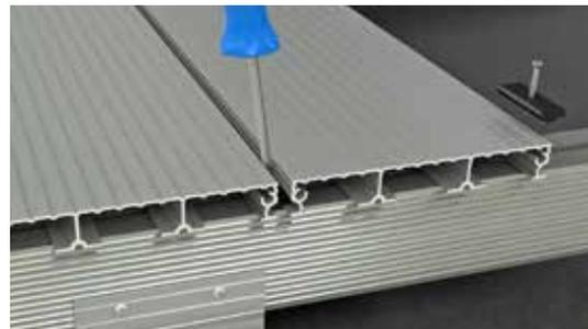
7. If the last board is not a full width. Fit the snap-on clip taking care to position it so that locates exactly between two "legs" of the aluminium boards. [use this image currently showing for 6. Cut the last board to fit (to edge of balcony or into doorways as necessary) using appropriate metal-cutting blades in suitable power tools.
