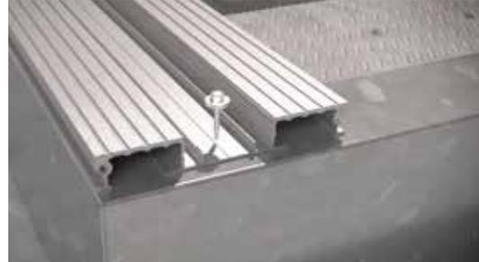
**NOTE:** Where boards are being fixed to a rigid substrate (for example a steel balcony) allowance must be made for thermal expansion by predrilling an 8mm hole in the base of the board at each fixing position, and leaving a min 3mm gap between board ends on runs in excess of 12 metres.
