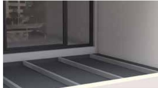
60 x 40mm **BoxRail™** rails should be spaced at maximum 600mm (950mm if using **Aspira**, 1000mm if using **Delta30**) apart with cleats spaced using the table below.
